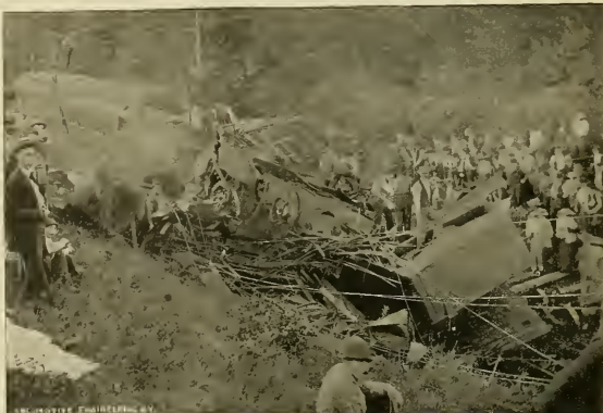
A HEAD-END VIEW OF THE FIRE BRICK AND IRON FRAME OF THE LOCOMOTIVE IN CENTER OF WORKS.
